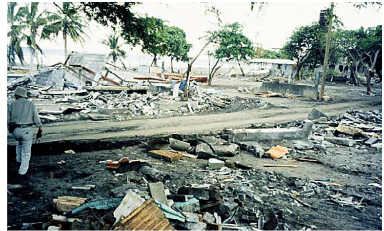
Damage from a tsunami
