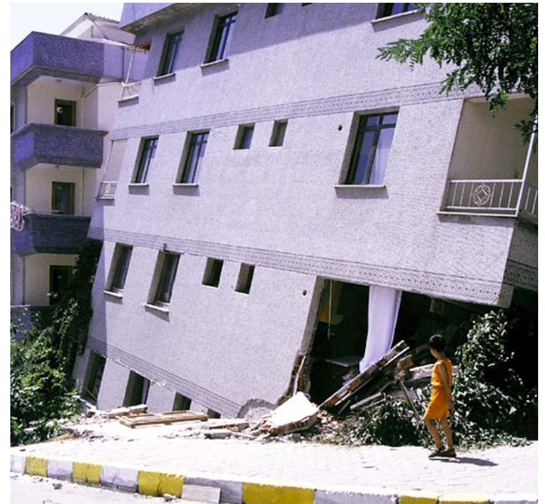
Earthquakes can damage or even destroy buildings.
