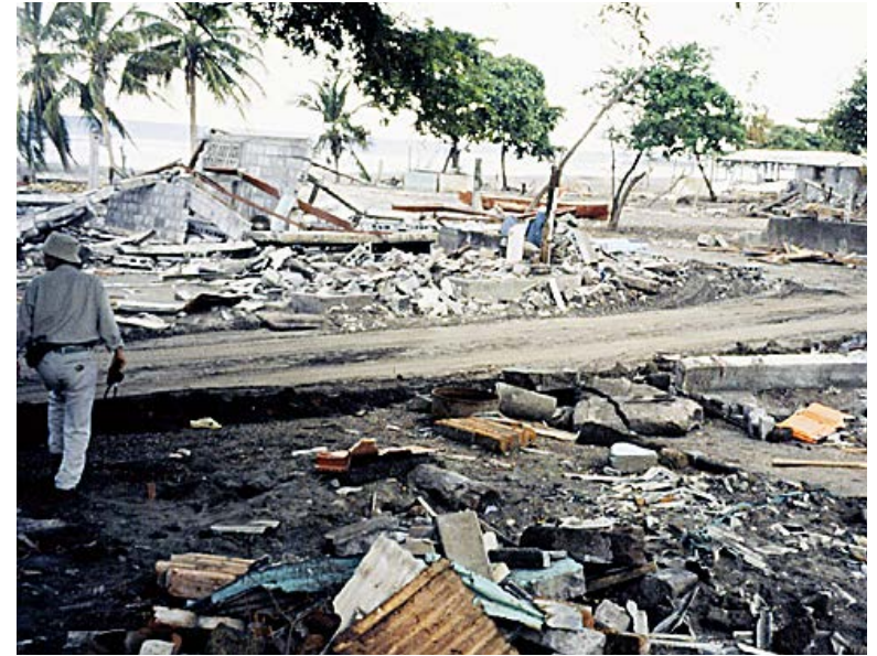
Damage from a tsunami
