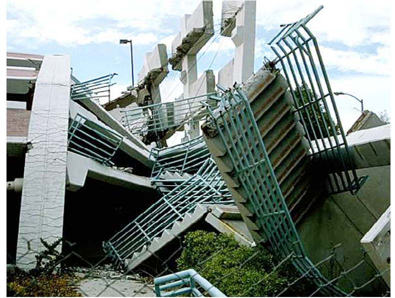
An earthquake destroyed this building.
