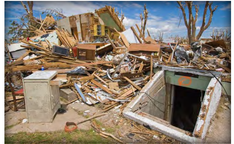
This underground shelter was built to provide protection from tornadoes, such as the one that destroyed the house next to the shelter.
